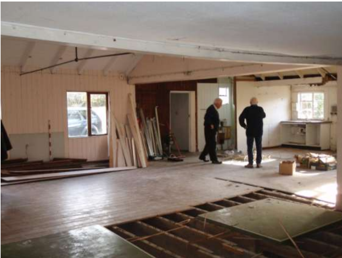
Plate 14. View of interior towards kitchen and toilet extension (Phase 2)
