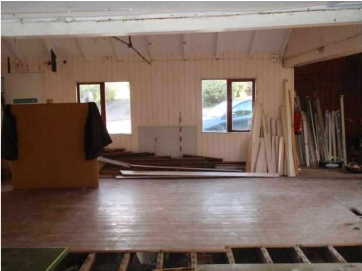
Plate 16. View of interior towards front of Phase 1 building
