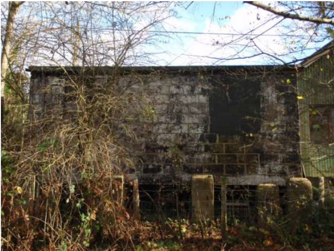
Plate 8. View of rear extension Phase 2 with blocked up windows (looking south-east)
