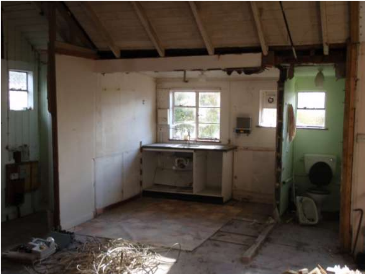
Plate 15. View of kitchen (Phase 2)
