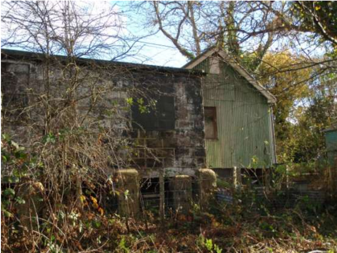
Plate 7. View of blocked up windows rear extension Phase 2 (looking south-east)
