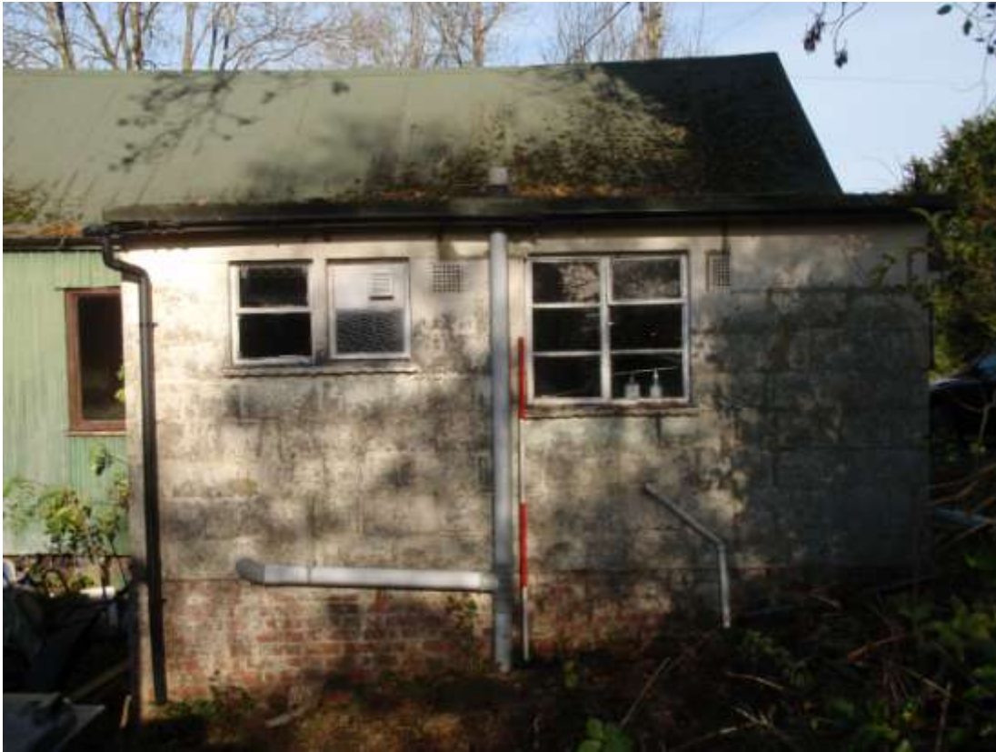
Plate 9. View of toilet and kitchen extension on brick base Phase 2 (looking north-east)
