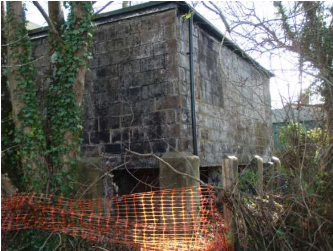
Plate 6. View of Phase 2 rear extension (looking south)
