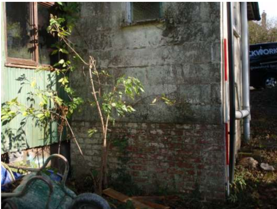
Plate 10. View of toilet and kitchen extension Phase 2 (looking north-east)
