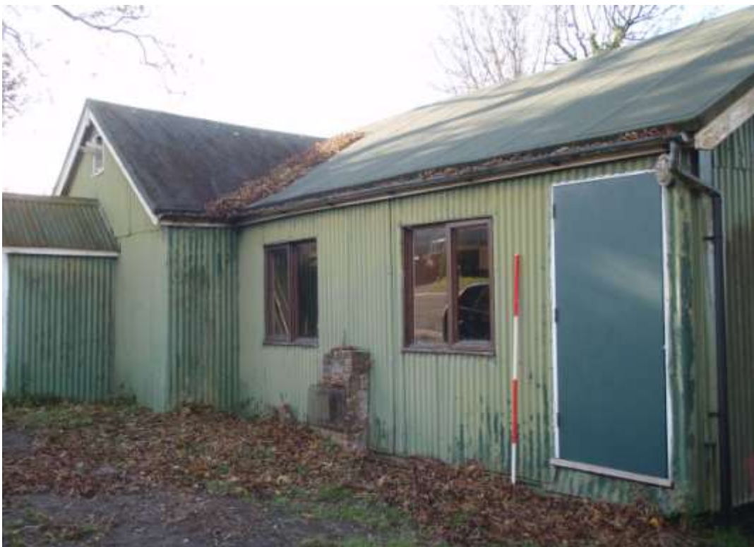
Plate 2. Front elevation (looking west)
