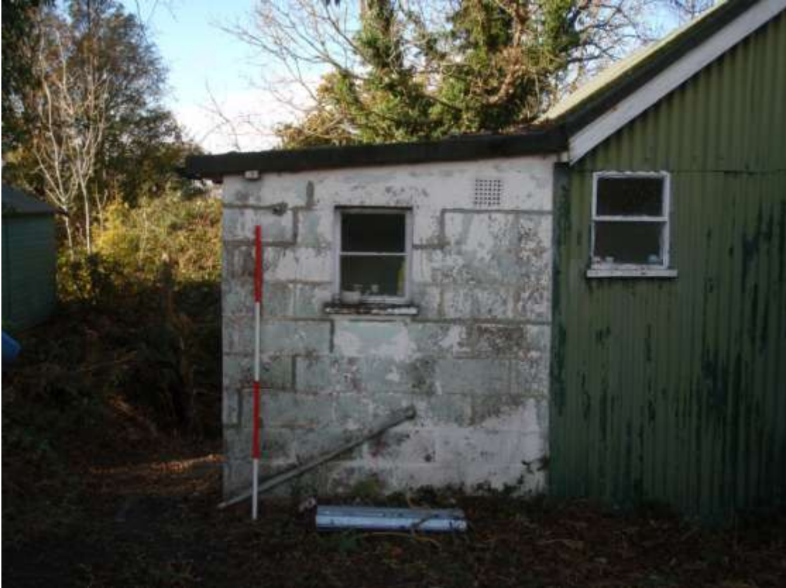
Plate 11. View of toilet and kitchen extension Phase 2 (looking north-west)
